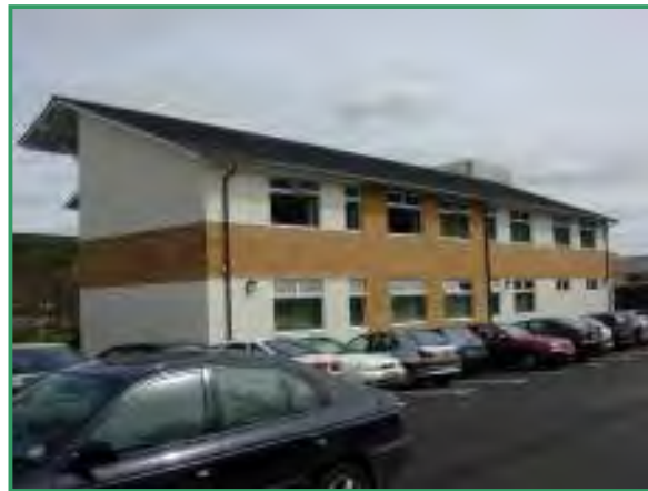
Above: At Tredegar Comprehensive School, a new teaching Block replaced poor quality temporary classrooms.
