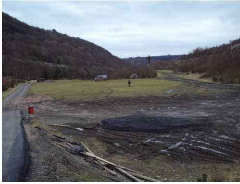
Plate 1: Six Bells site looking south from northern boundary
