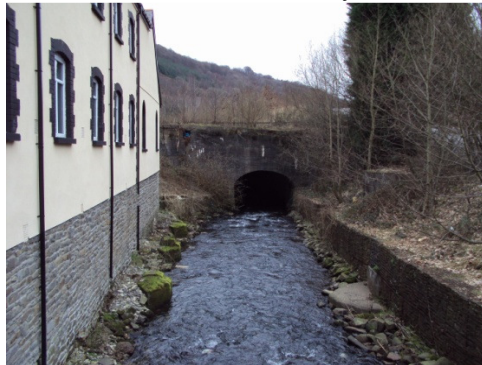
Plate 3: Ebbw Fach River and culvert, looking downstream (south). The building on the left is the Six Bells Baptist Church
