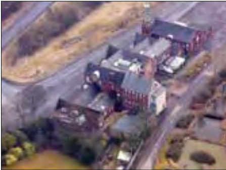
8. General Offices from the north west
