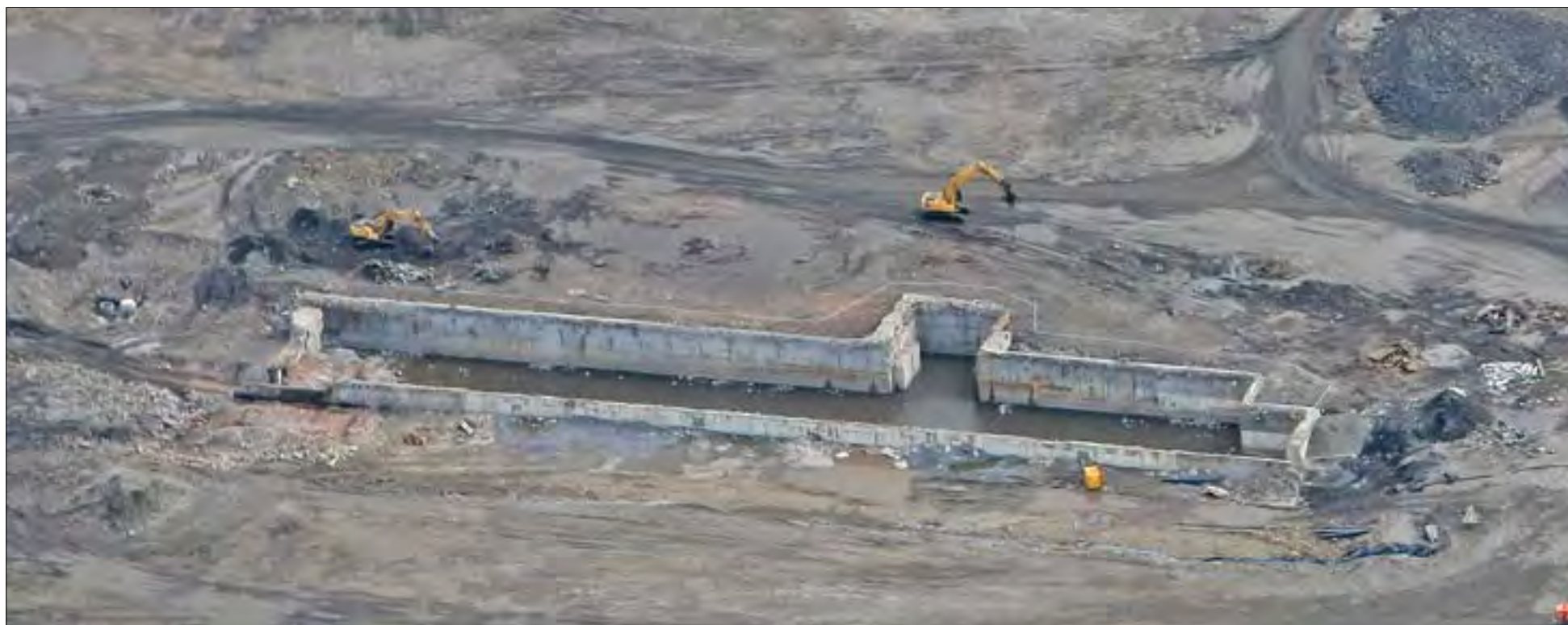
Figure 26: ETL 4 during reclamation
