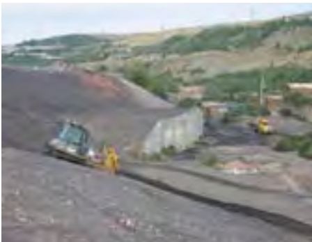
Figure 13: Images of the site undergoing reclamation
