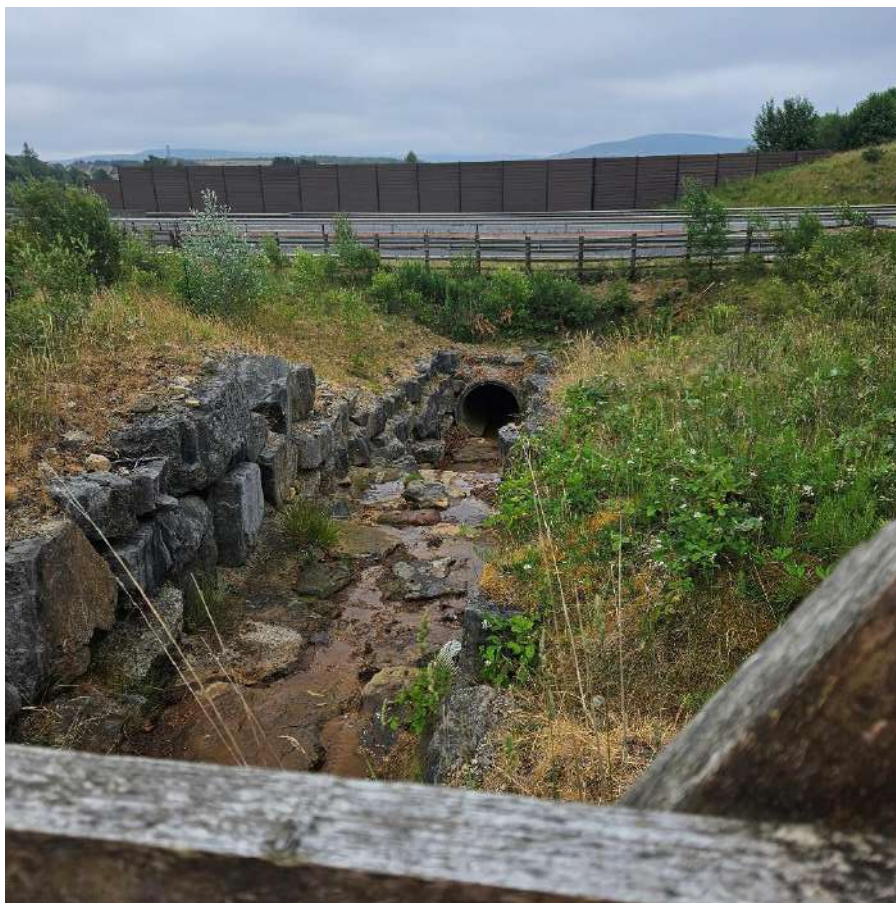
Figure 6: East facing view of A465 and drainage culvert fed by artificial ditch.
