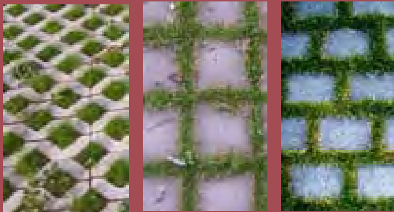
Although not appropriate for every location, permeable paving in car parks can reduce the amount of water runoff considerably and make the infiltration process as local and direct as possible
