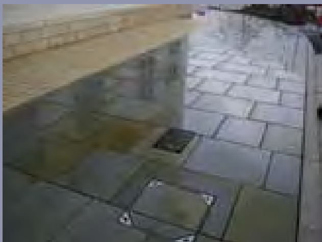
This surface blends a number of different materials. Cuts and patterns are very simple and service covers have been well integrated.
