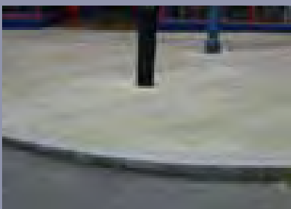
Top Image: Cutting straight road kerbs to suit tight radii at Brynmawr
