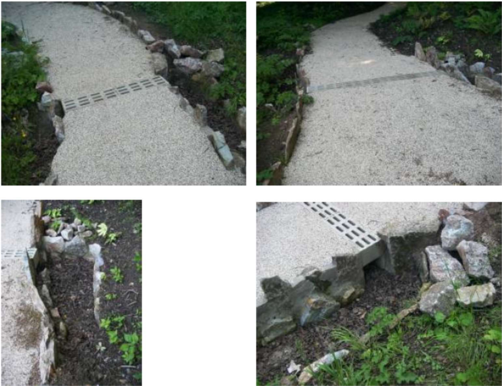
'Aco 300' GCN tunnel sections with custom stone-built headwalls, used on footpaths
