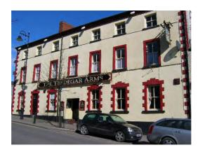
**Photo 6.13:** The Tredegar Arms has retained its attractive "traditional" patterns of fenestration (usually with glazing bars/transoms and mullions set back within a reveal) and consistent floor-to-ceiling heights (usually in diminishing proportions from the ground storey upwards.
