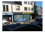
Photo 6.5: Examples of insensitively designed shop fronts on Castle Street – although the shop front on the far right has retained its pilasters, stallriser and angled fascia.
