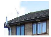
Photo 5.17: Concrete interlocking roof tiles and terracotta ridge tiles (as shown on this modern infill building on Elim Court, Upper Salisbury Street) are not appropriate.
