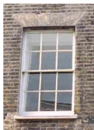
Photo 5.21: Example of a timber sash window (not in Tredegar) with stone lintel above, glazing separated by timber mullions and transoms.
