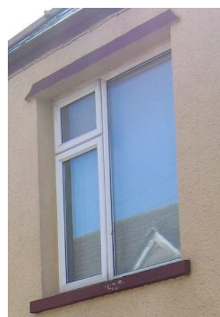
Photo 5.20: Example of a typical insensitively designed standard UPVC window in Tredegar, which has replaced an original sash window.
