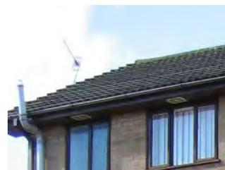
**Photo 5.17:** Concrete interlocking roof tiles and terracotta ridge tiles (as shown on this modern infill building on Elim Court, Upper Salisbury Street) are not appropriate.
