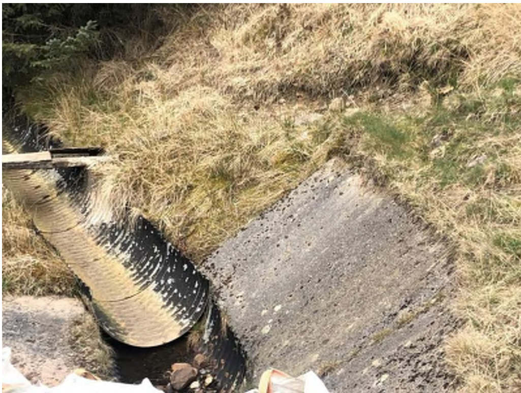
Perimeter drainage ditch (lined with concrete and corrugated metal).
